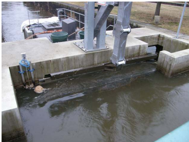
Abb. 177: WKA Plaue (Rechen + Bypass)
